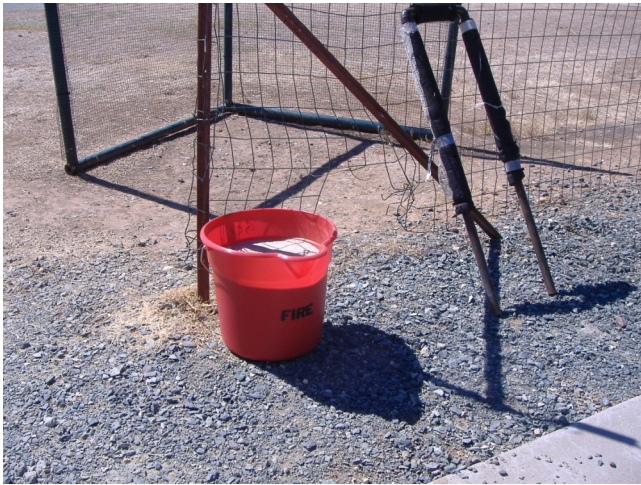
Portable sand buckets at the openings in the fence going to the runway.
